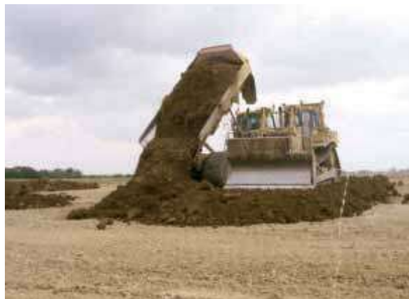
Starting a 'peninsula' of topsoil
