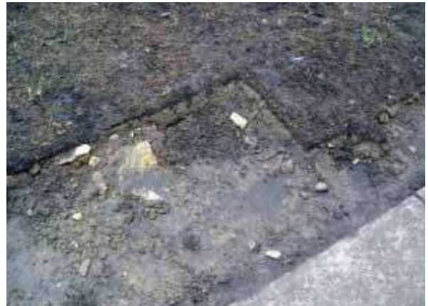
Surface water running onto adjacent paving
