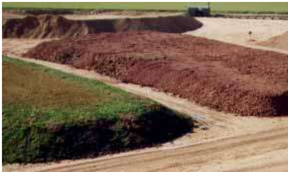
Clearly defined stockpiling of different soil materials
