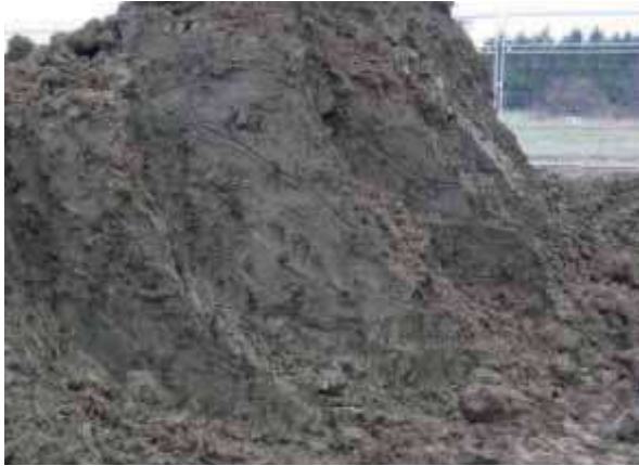
Topsoil stockpiled when wet and plastic
