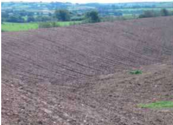
Permanent storage created for surplus topsoil stripped from a greenfield site in Devon, despite there being demand for topsoil in the locality.
